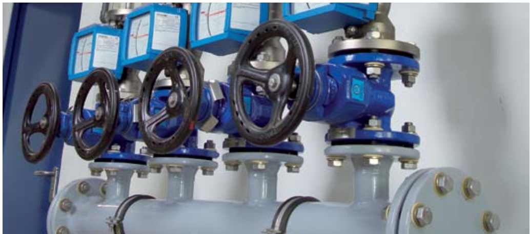
Drinking water treatment plant Luisenthal, Germany VAG BETA 200 Gate Valves
