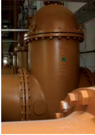
Cologne combined pumping station Rodenkirchen, Germany VAG KOS Gate Valves
