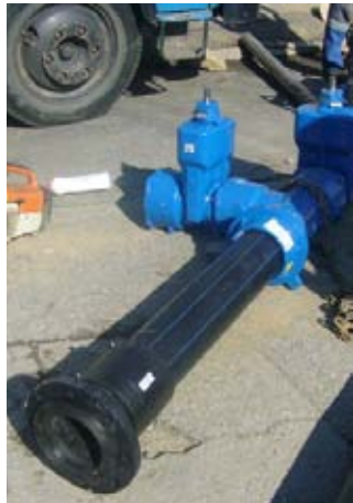
Refurbishment of the water supply network in Ždár, Slovak Republic VAG BAIO BETA 200 Gate Valves
